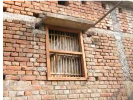
Figure 6: Brick and cement mortar
