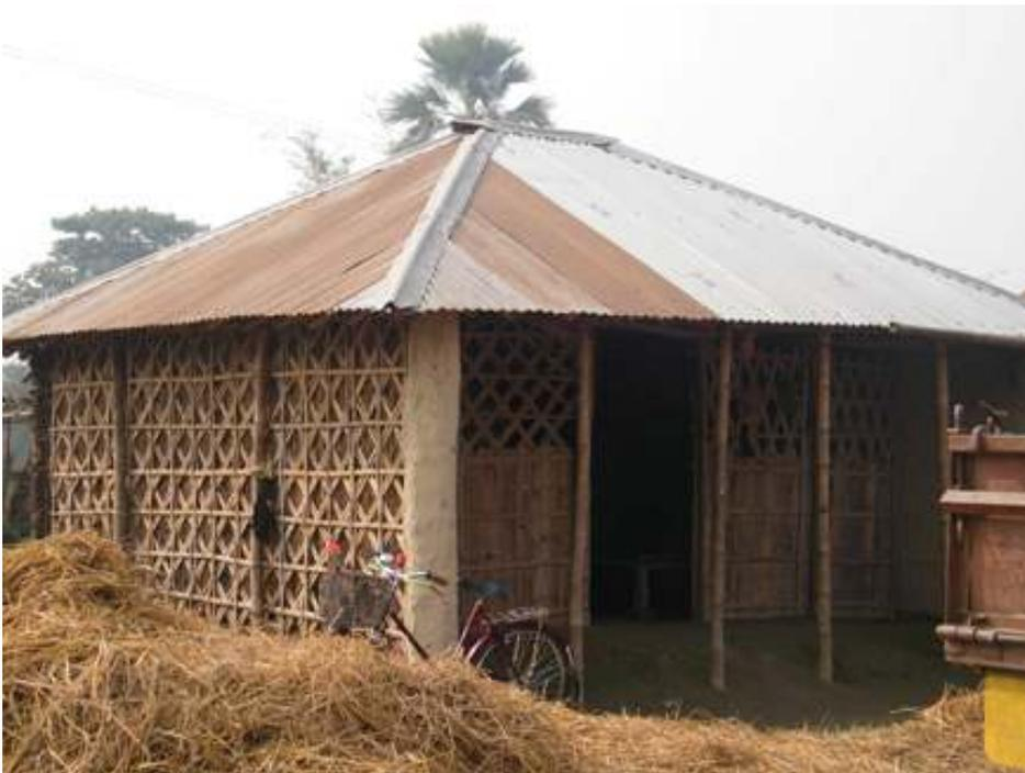
A ‘fusion’ house built by an affected family themselves. Gi-sheet roof, bamboo jaali and bamboo slats walls, cement ‘columns’, bamboo pillars, bamboo roof structure
