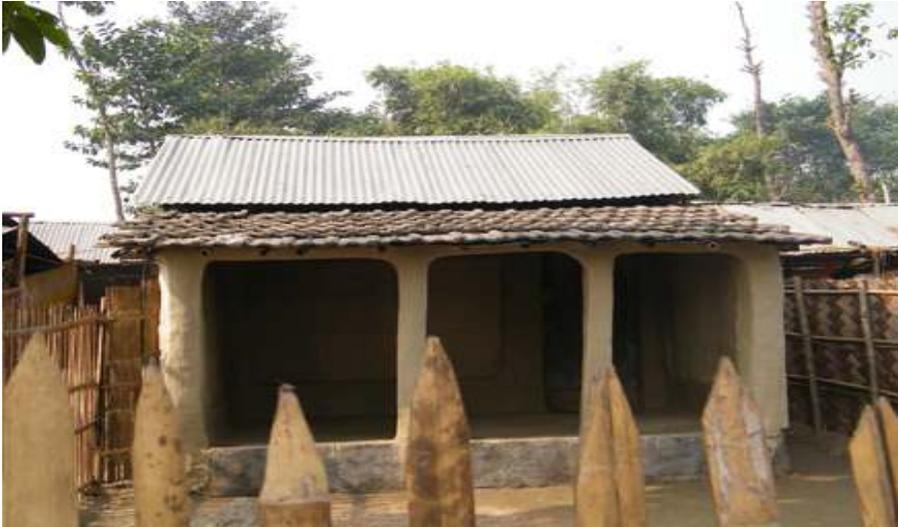
A fusion house: tile-roof verandah; GI-sheet roof for main house, mud walls, bamboo roof structure. A lot of the materials are recycled materials retrieved from the old damaged house.
