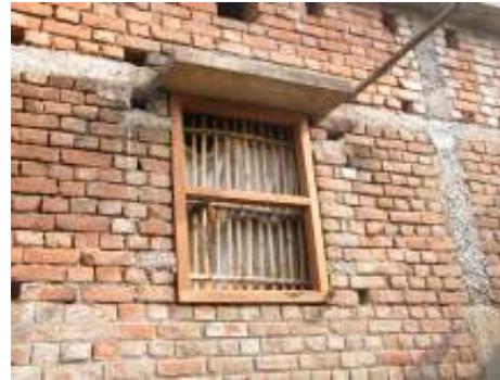
Figure 6: Brick and cement mortar
