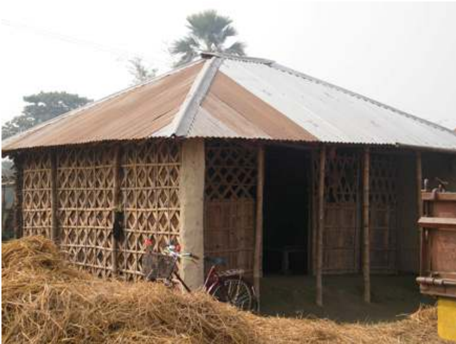
A ‘fusion’ house built by an affected family themselves. Gi-sheet roof, bamboo jaali and bamboo slats walls, cement ‘columns’, bamboo pillars, bamboo roof structure - Mirgunj, Madhepura District, Bihar
