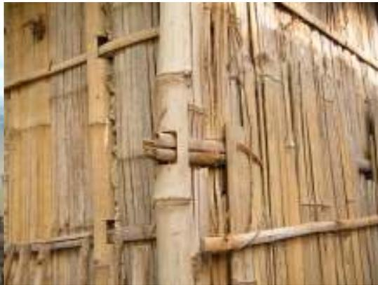
Figure 13: Bamboo joineries
