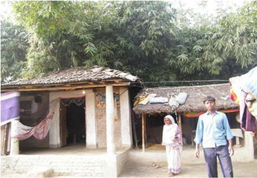
An Indira Awas Yojana house of brick and cement, tile with bamboo roof structure, cement columns and a mud-thatch-bamboo sleeping quarters as an additional room.
