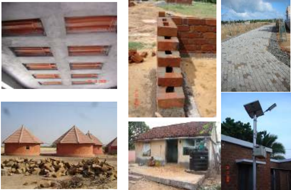
Filler-slab roof, rat-trap bond walling, permeable roads and drains (water management), 'pucca' brick and tile bhungas, rain-water harvesting, solar street lights.
