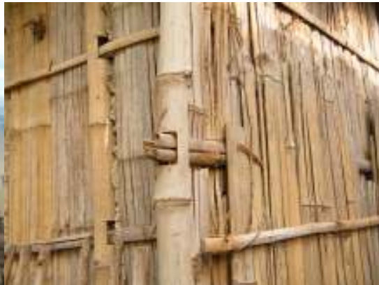
Figure 13: Bamboo joineries
